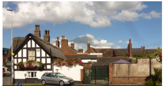
Rear of the White Bear Inn, room now demolished
